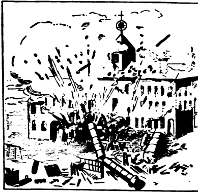
FIG. 164.—BOILER-EXPLOSION AT DAYTON, OHIO.
